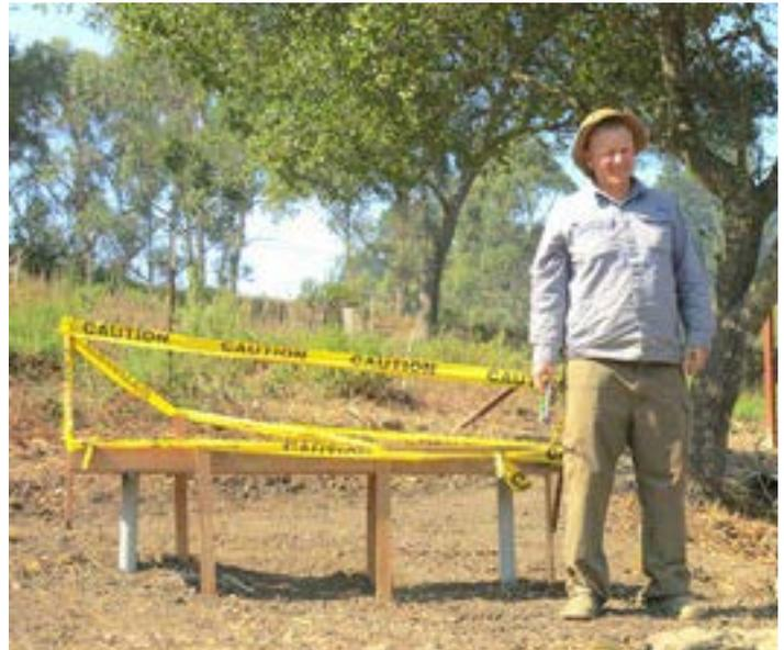
Here is Matt with that part all done, the bench still braced and taped to let the concrete cure.
