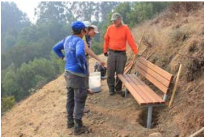
Here's the first bench going in at Diablo Bend. We dug the post holes with a rock bar and post-hole digger. It was tough going. You can see it's not quite set in this shot. The wood for this bench came from the old sideboards of my daughters' sand box. Soon, we mixed and poured concrete around the posts and braced and all wrapped up in yellow tape. It was so smoky there that we couldn't even see Mt. Diablo but we got the perfect placement anyway!
